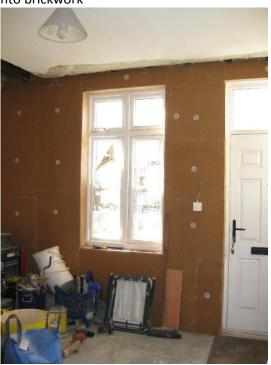
Insulation was continuous through floor void, which entailed cutting out floorboards and ceiling plasterboard to accommodate it.
