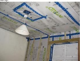
Naidec (black double-sided sticky tape) was used prior to service zone batons being fixed, in order to maintain airtightness after the drill had created a hole for the concrete screw.
