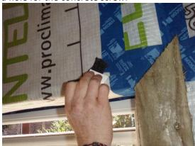
The stud wall next to one of the bedrooms opened directly into loft, so this had to be trimmed off in order to allow the membrane to pass in a continuous layer from the external wall through to the solid partition wall next to the stairs.
